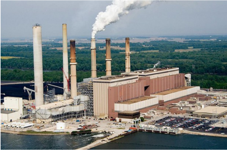
Fig. 3 Duke Energy facility
